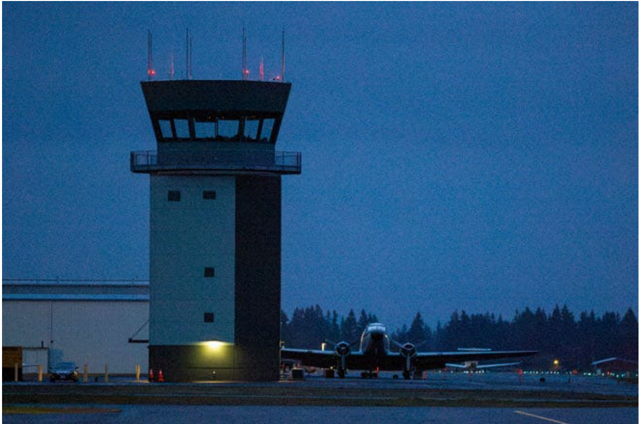
Air Traffic Control Tower at Aurora State Airport. Kevin Neri, Statesman Journal
